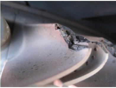
Figure No.19 Broken edges on first stage turbine bucket.
