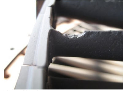
Figure No.22 Signs of dents and broken metals on second stage turbine bucket.
