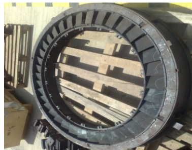
Figure No.14 Signs of burnout on first stage turbine nozzles.
