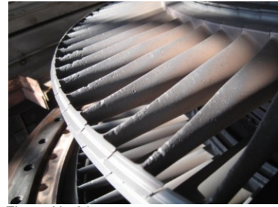
Figure No.21 Signs of dents and broken metals on second stage turbine bucket.
