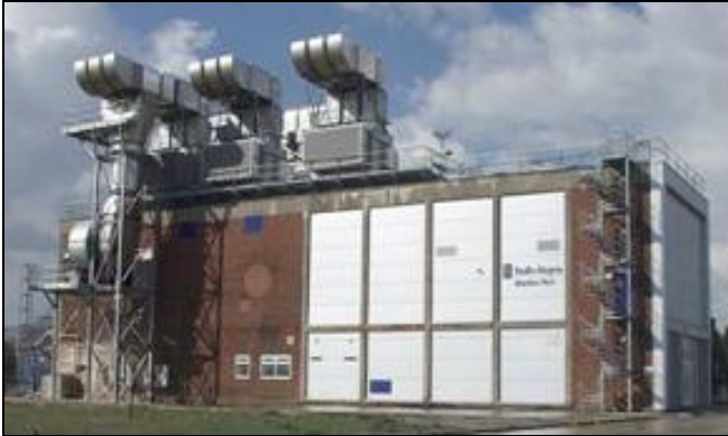
FIGURE 3- MT30 TEST BED, BRISTOL UK (SHOWING LOAD BANKS AND HEATED AIR INTAKE)
