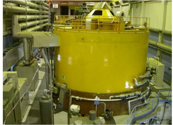
Figure 5. 70 MVA - 10 kV generator of the first 67.5 MW - 50 Hz unit running at 500 rpm.
