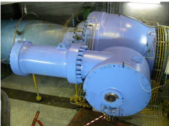
Figure 4. Ball valve at the end of each penstock.
